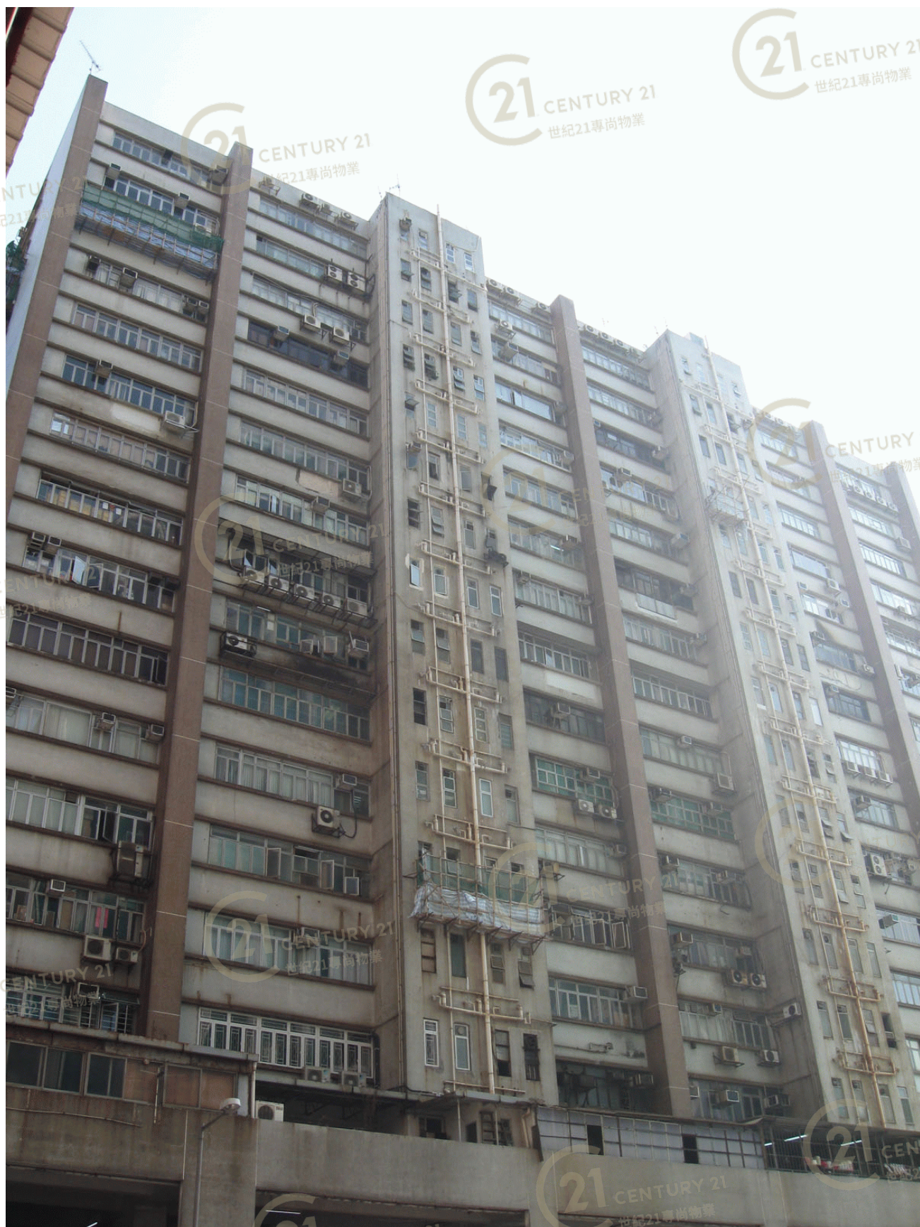
永恒工業大廈 Wing Hang Industrial Building
