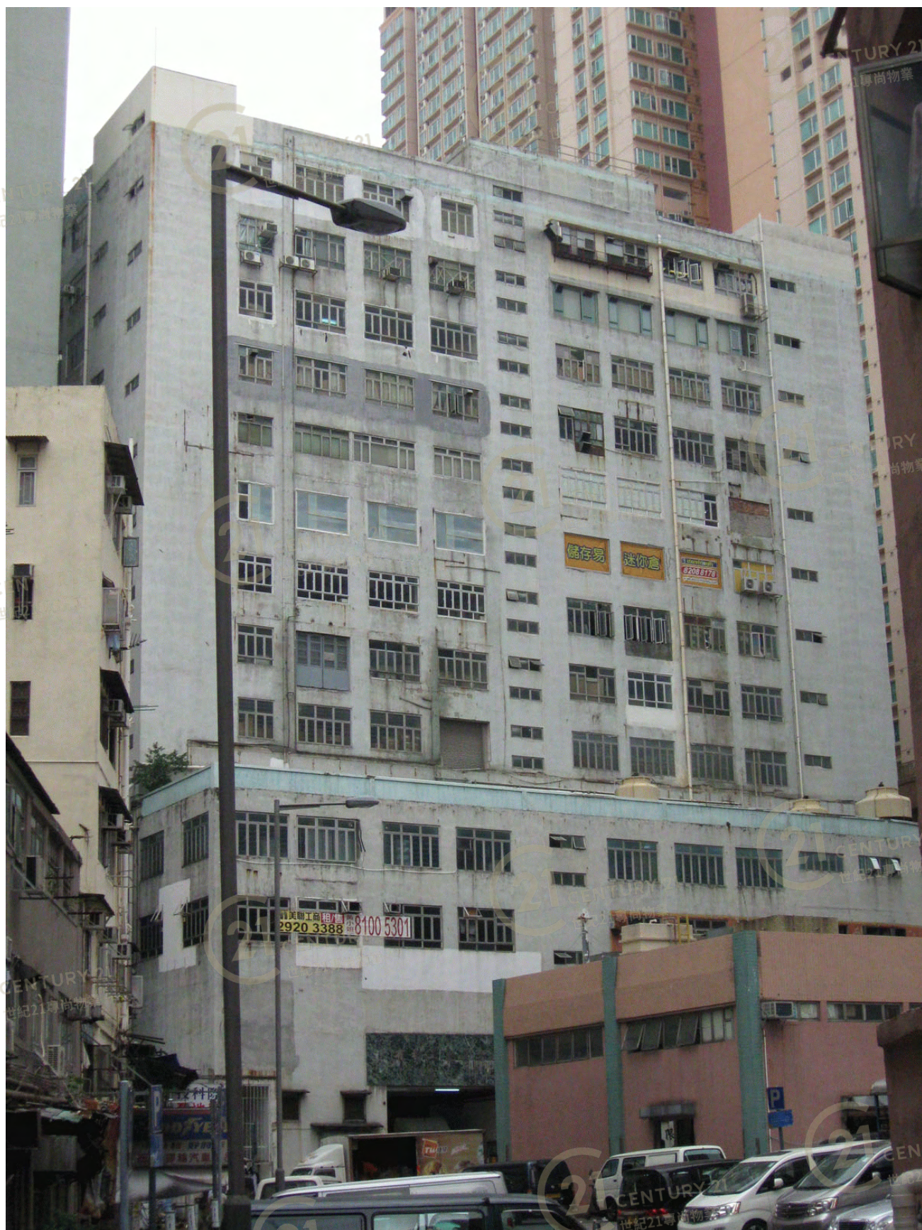
有利工業貨倉大廈 Mercantile Ind & Warehouse Building
