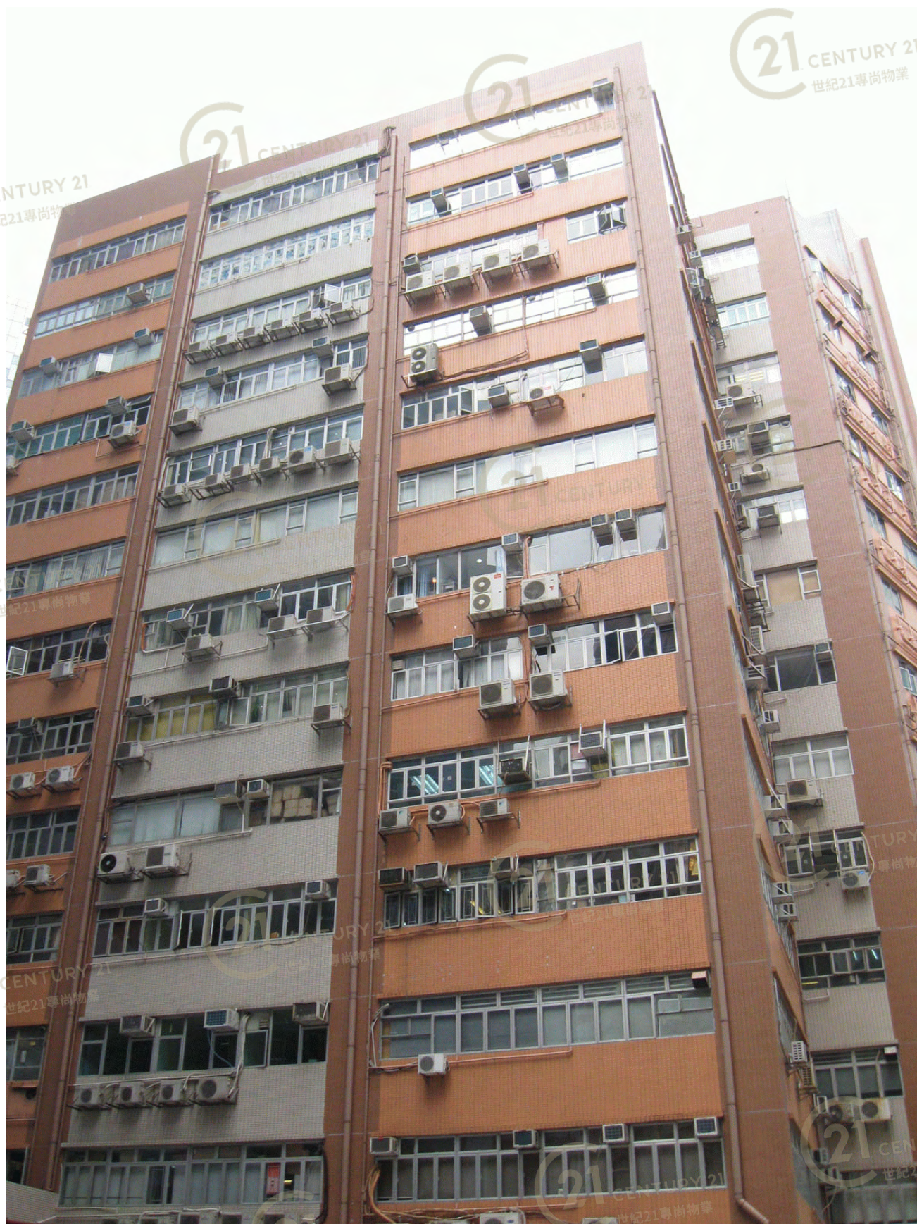
力豐工業大廈 Effort Industrial Building
