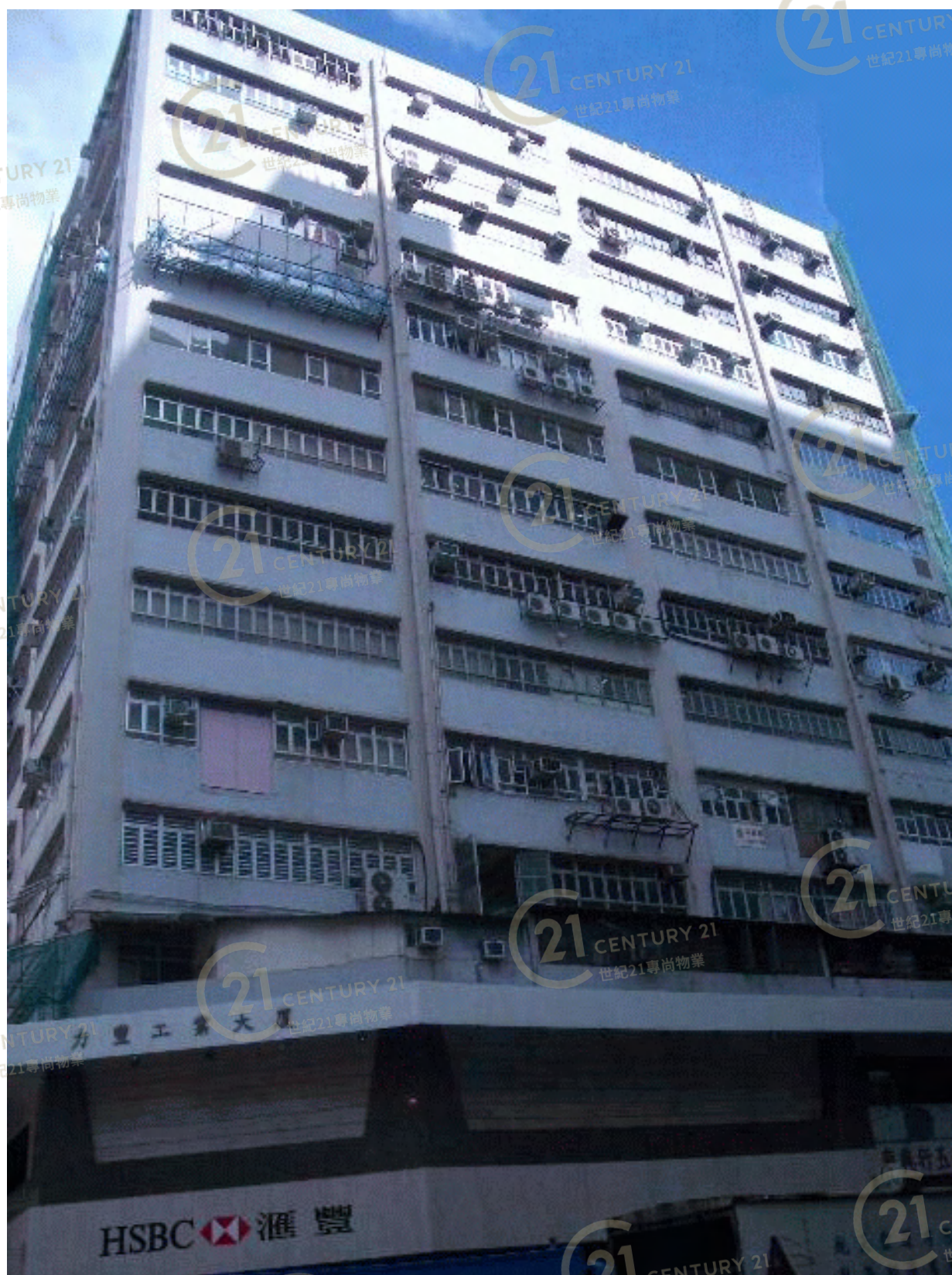
力豐工業大廈 Effort Industrial Building
