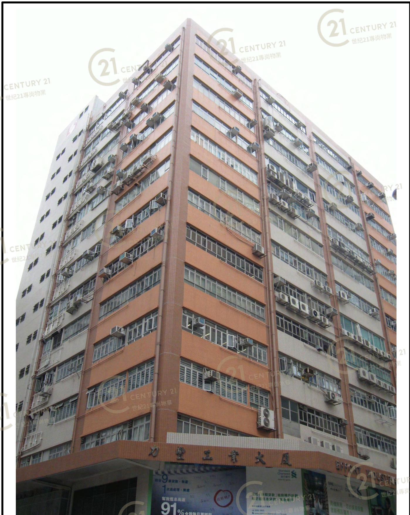
力豐工業大廈 Effort Industrial Building
