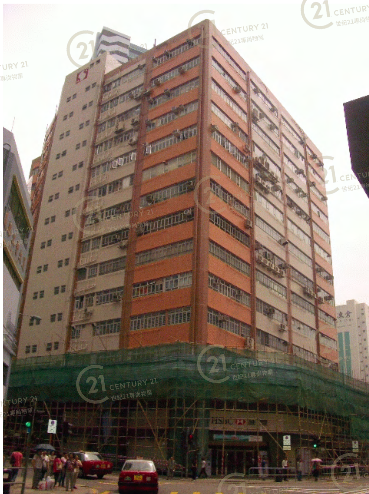
力豐工業大廈 Effort Industrial Building
