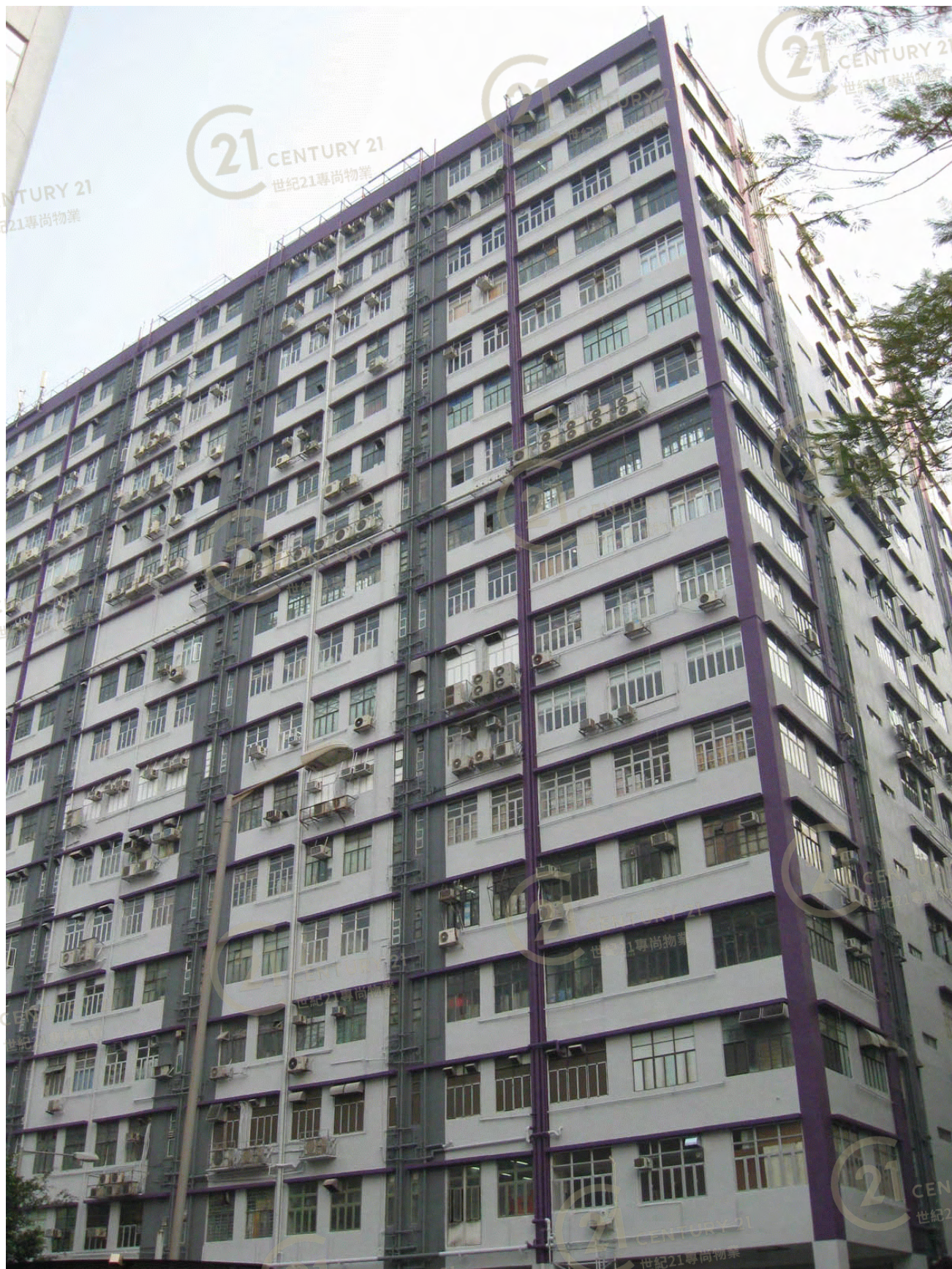
華生工業大廈 Wah Sang Industrial Building
