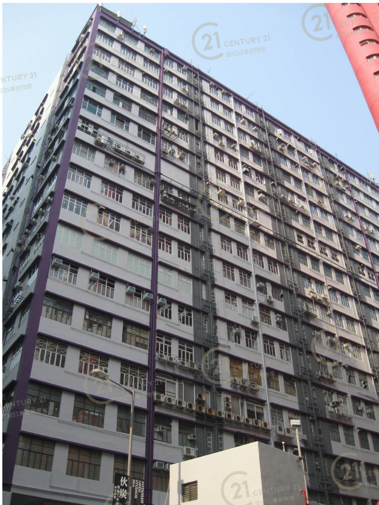
華生工業大廈 Wah Sang Industrial Building
