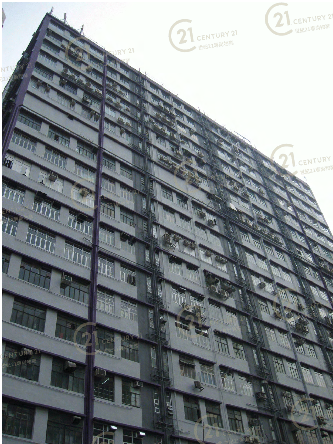
華生工業大廈 Wah Sang Industrial Building
