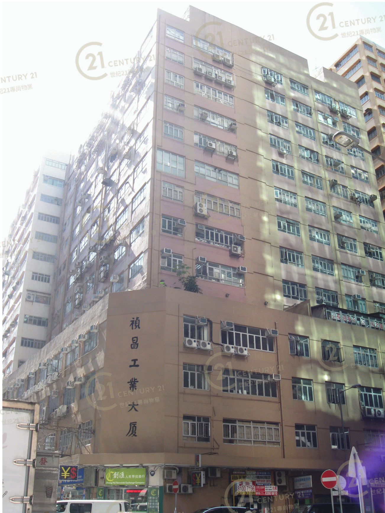
禎昌工業大廈 Ching Cheong Industrial Building
