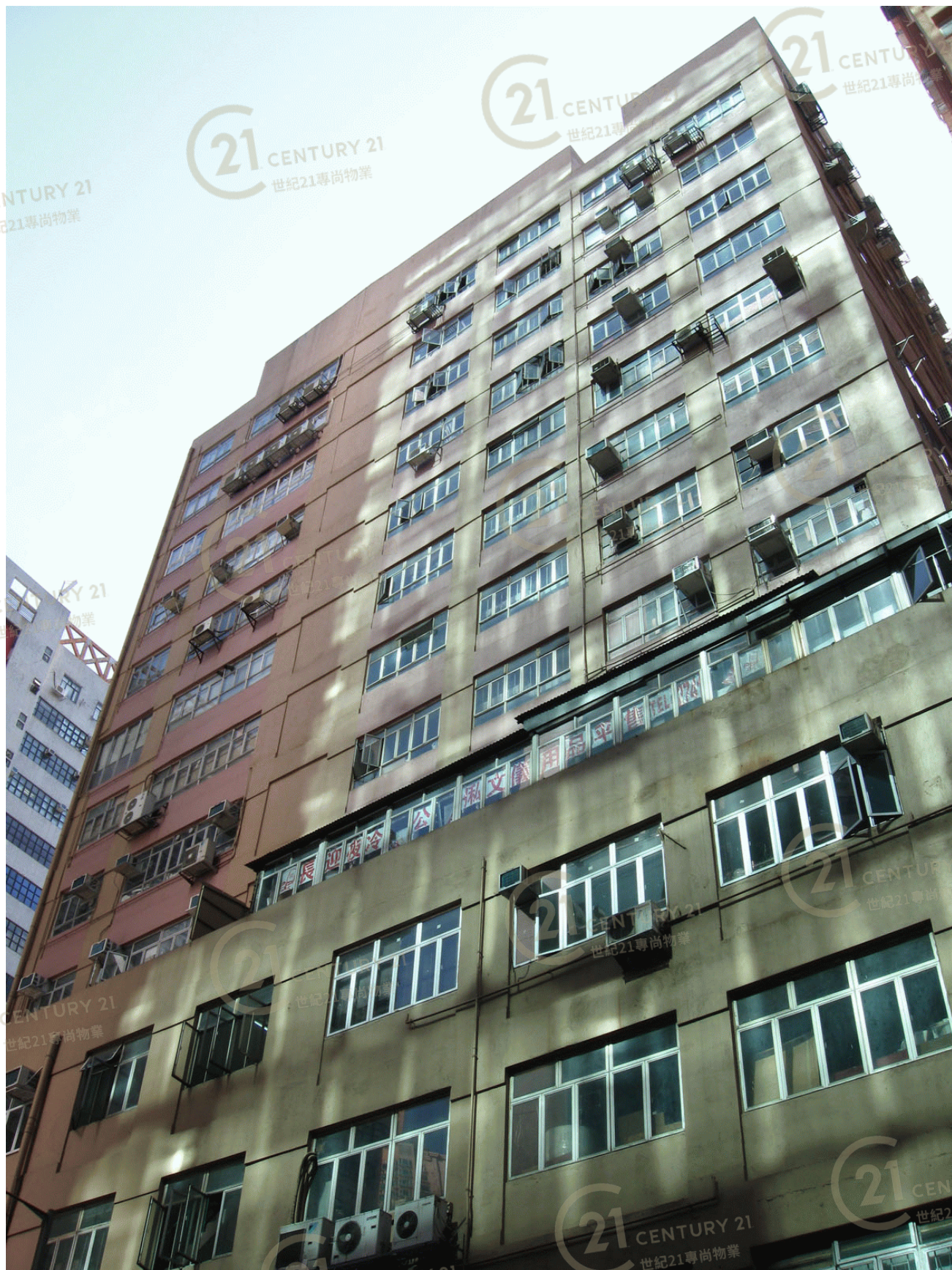
禎昌工業大廈 Ching Cheong Industrial Building
