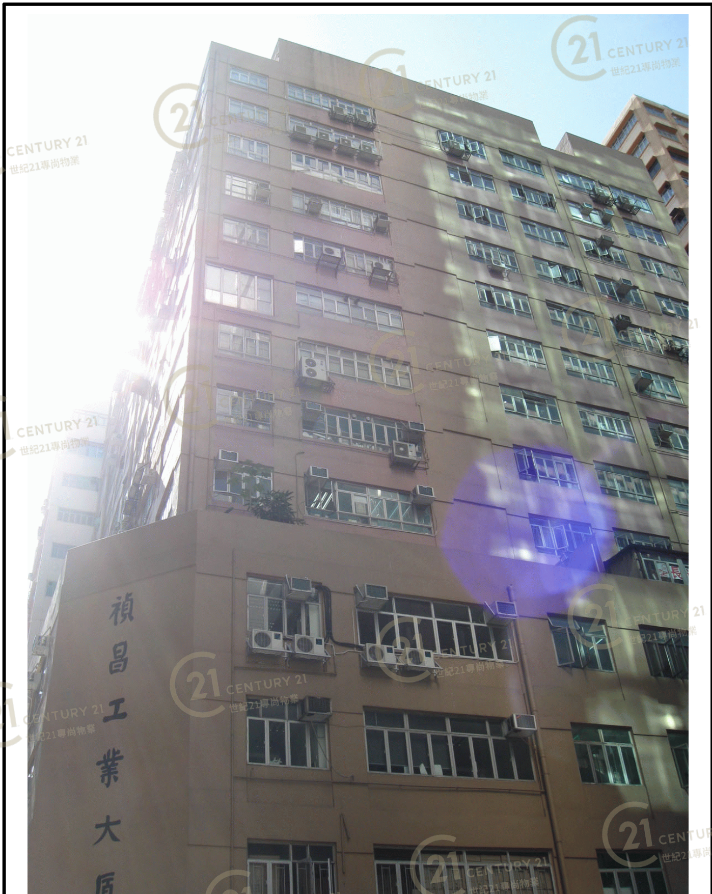
禎昌工業大廈 Ching Cheong Industrial Building
