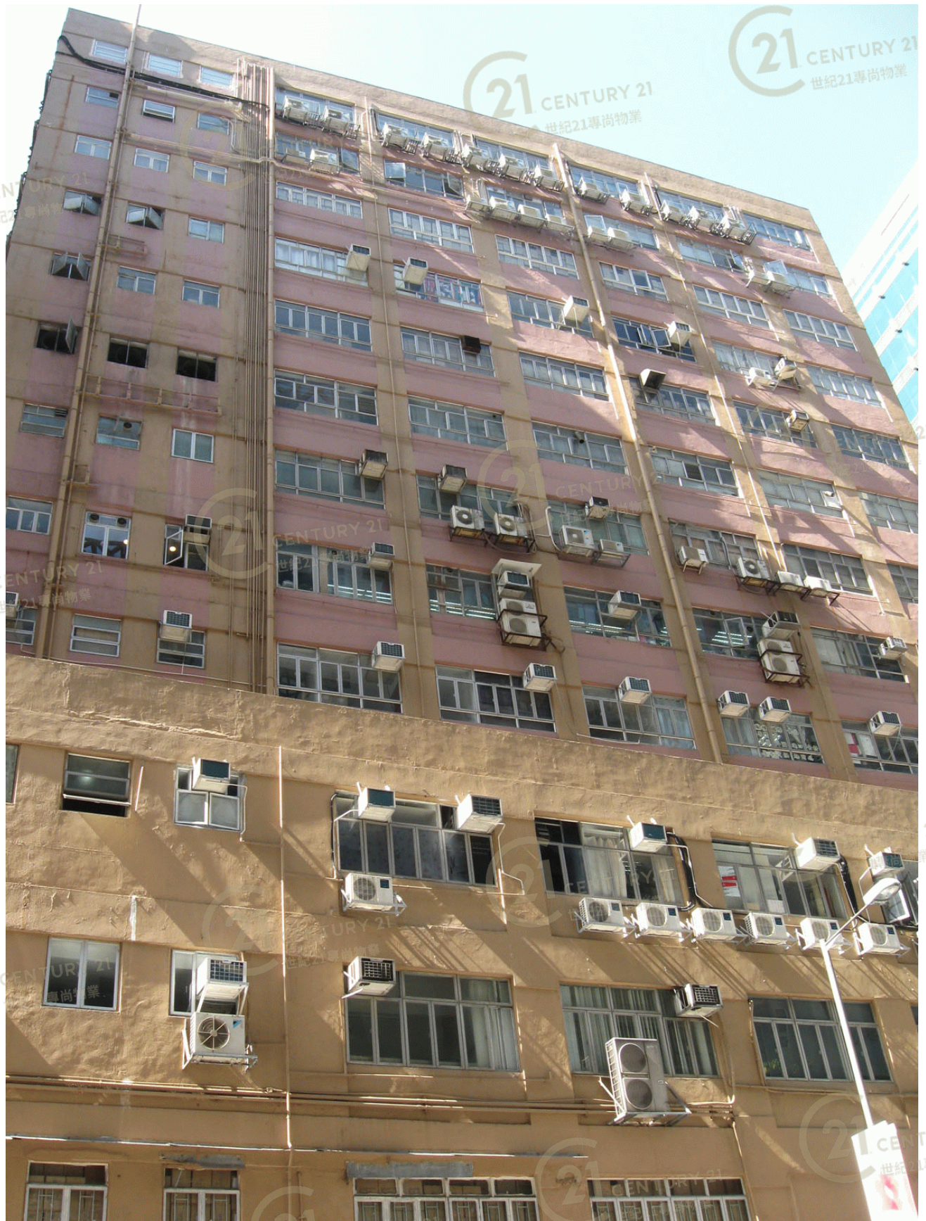
禎昌工業大廈 Ching Cheong Industrial Building
