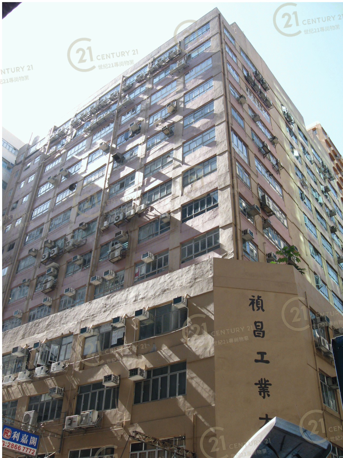
禎昌工業大廈 Ching Cheong Industrial Building
