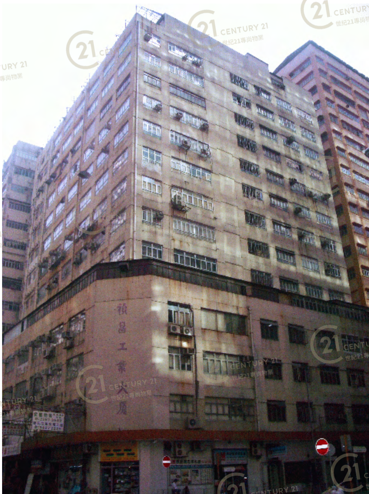
禎昌工業大廈 Ching Cheong Industrial Building
