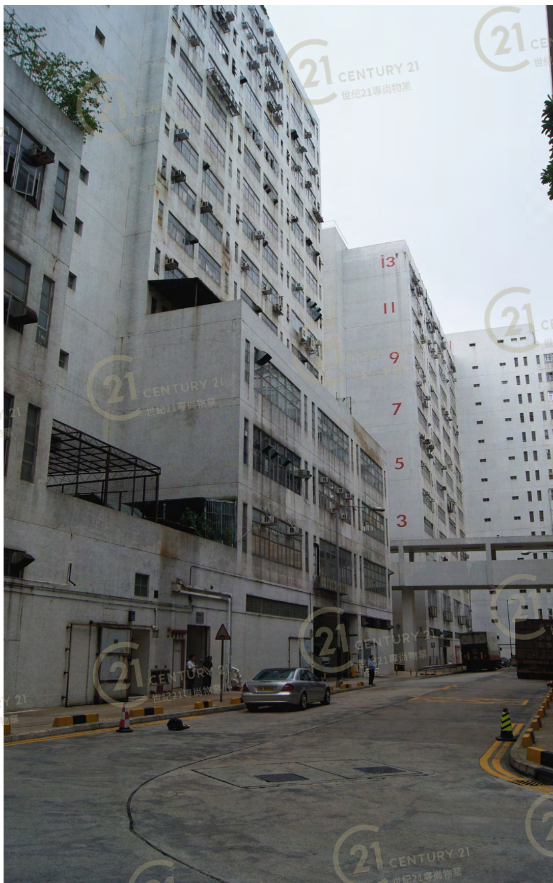
南豐工業城2座 Nan Fung Industrial City Block 2
