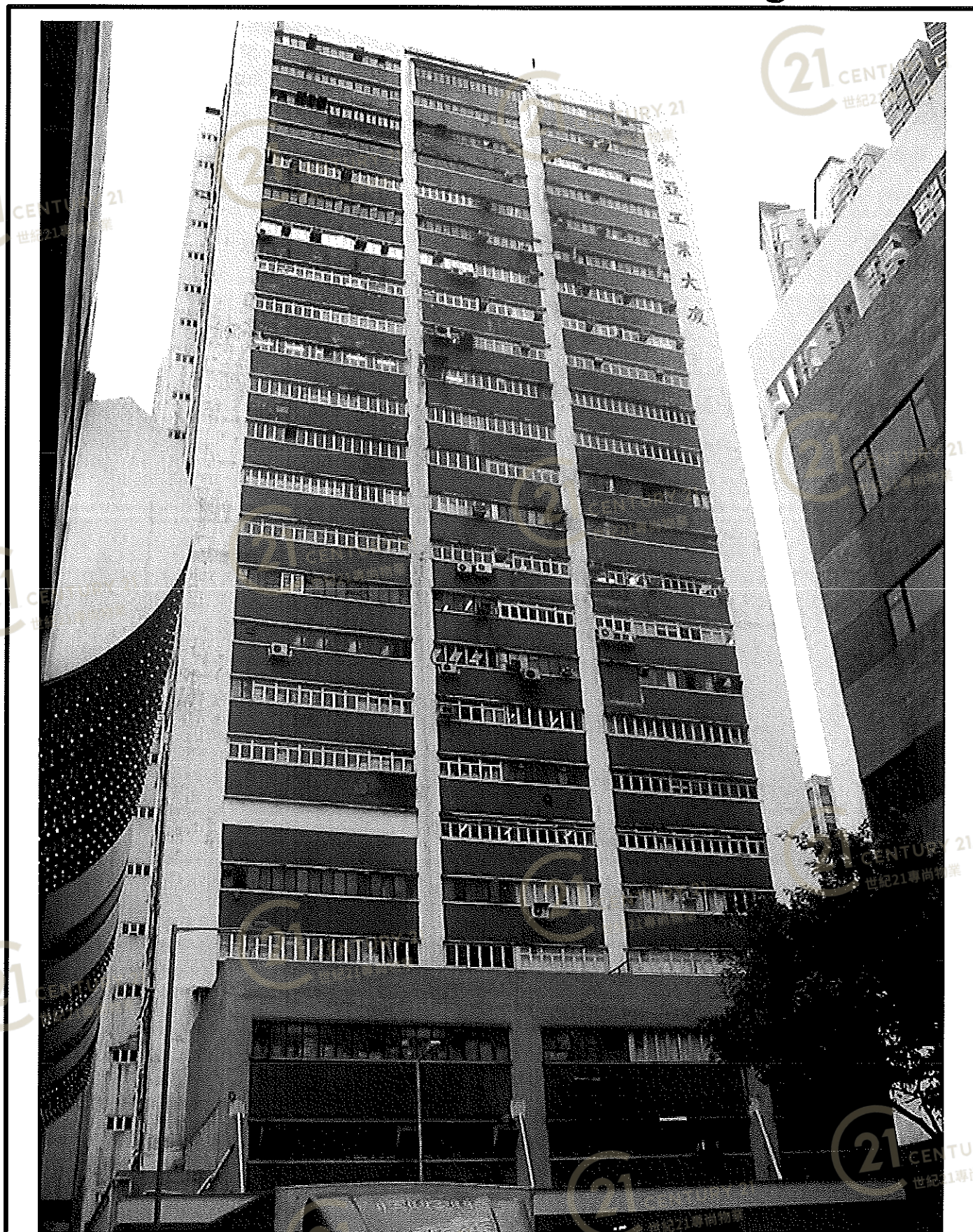
榮亞工業中心 Young Ya Industrial Building
