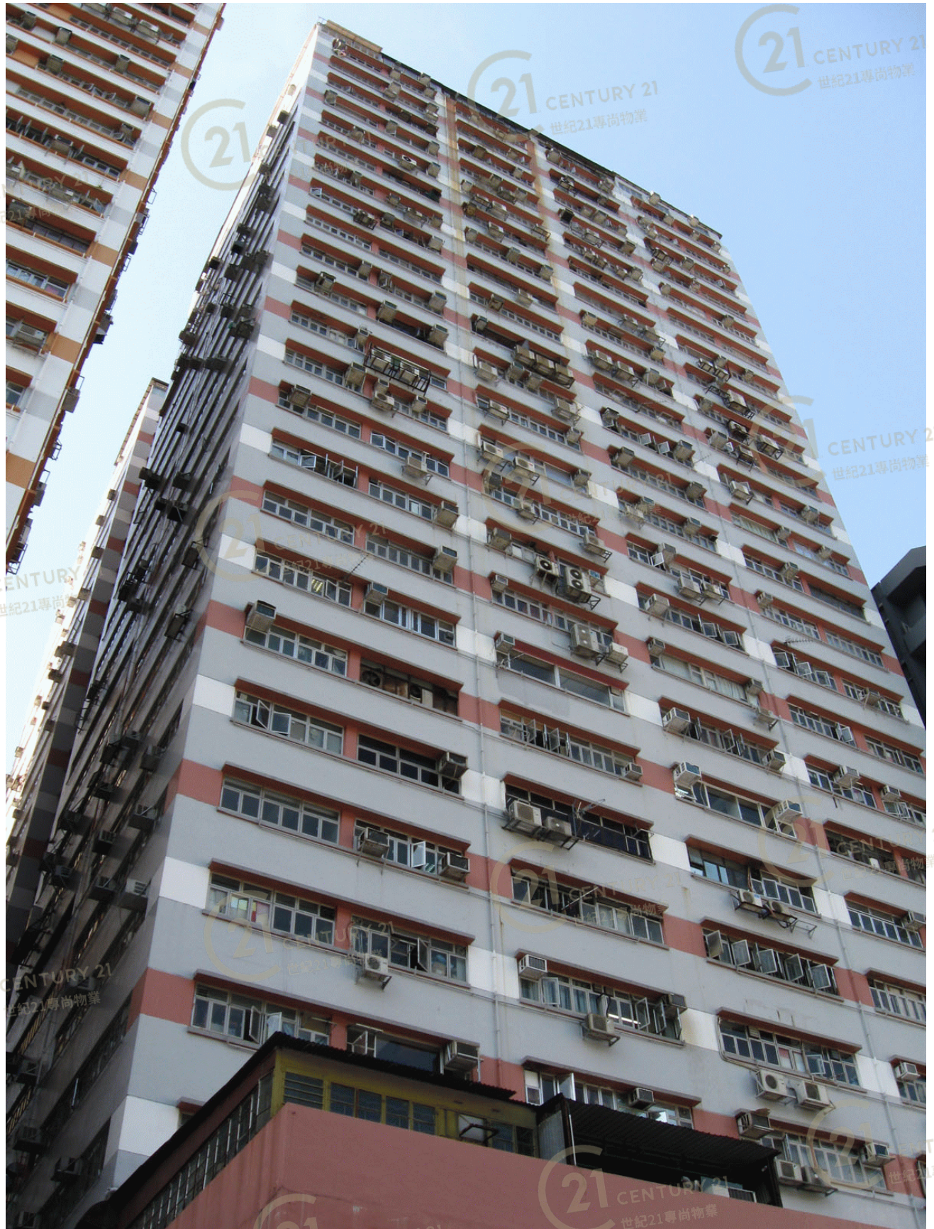
金豐工業大廈1座 Goldfield Industrial Building Block 1
