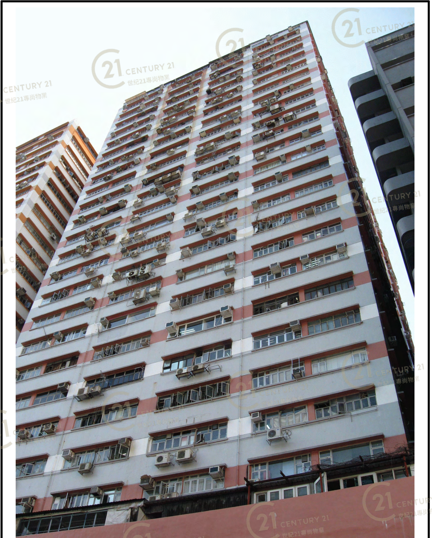
金豐工業大廈1座 Goldfield Industrial Building Block 1
