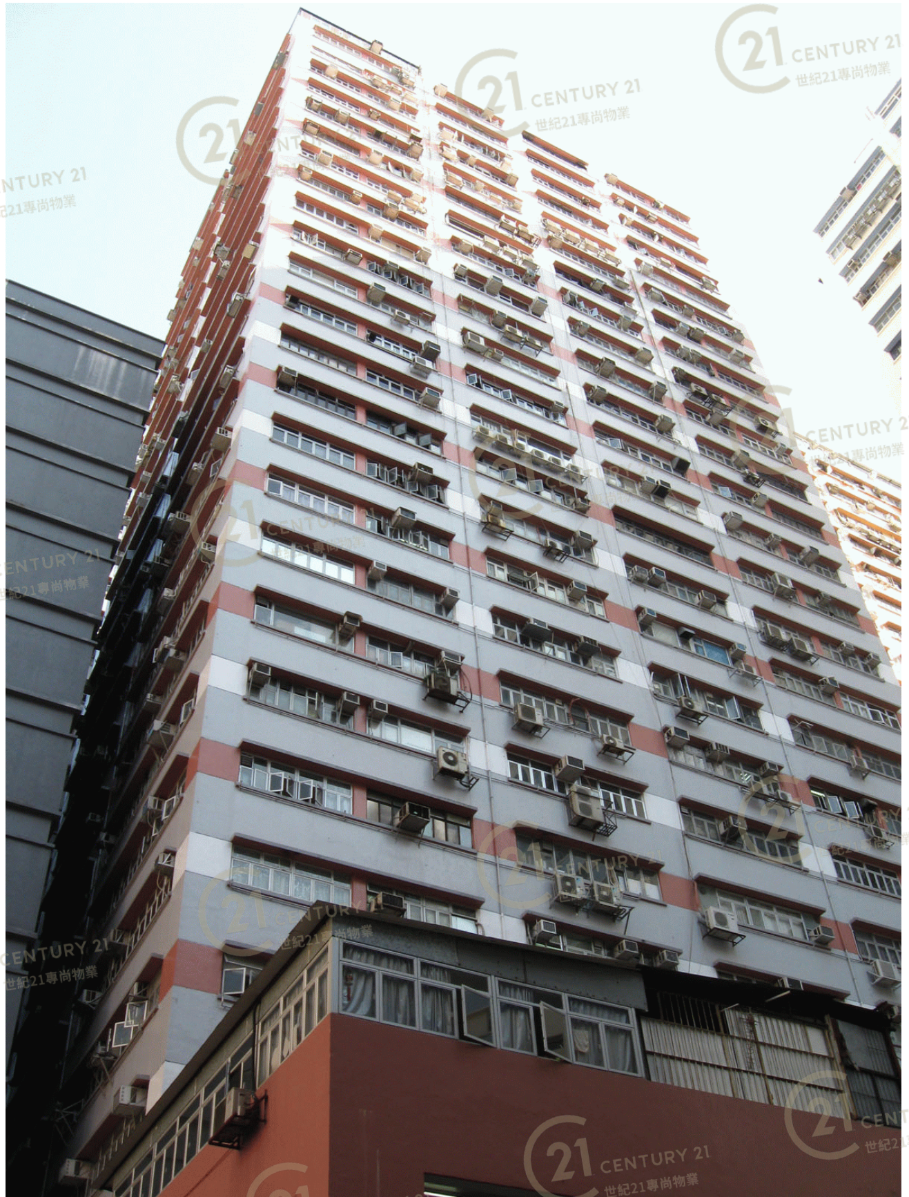
金豐工業大廈1座 Goldfield Industrial Building Block 1
